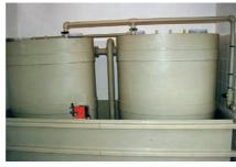
the strictest criteria. The special double jacket version replaces also an emergency tank. Fitted with other accessories (stirrers, pumps, dosing devices for powder substrates) they become full-fledged units for preparation of chemical solutions. It is recommended to install a reservoir on a flat base slab.
